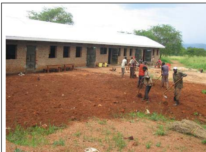
All outside doors are fitted and community at work.
