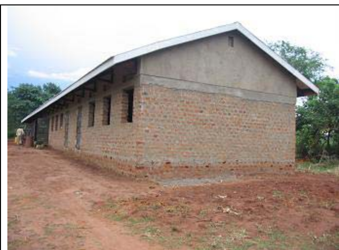
Side view after facia board and plastering (Current)
